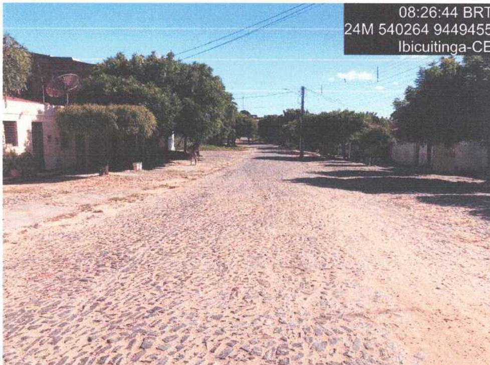
Figura 286 – Rua MELQUIADES ALVES MAIA (FINAL)
